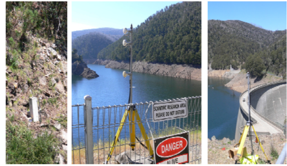
Figure 8: Locata receiver installation at Tumut Pond Dam
