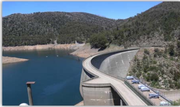
Figure 7: Tumut Pond Dam (Total View)
